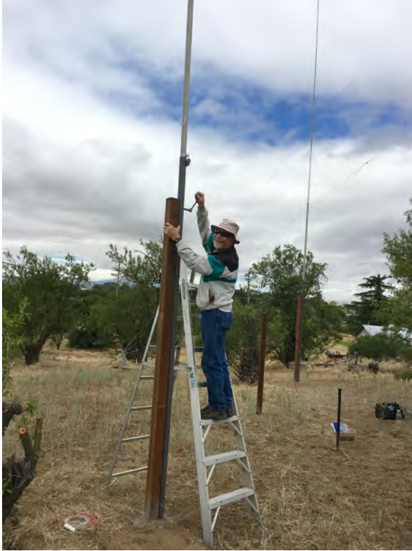
Figure 3. WB6ETY bolts the East element into place.
