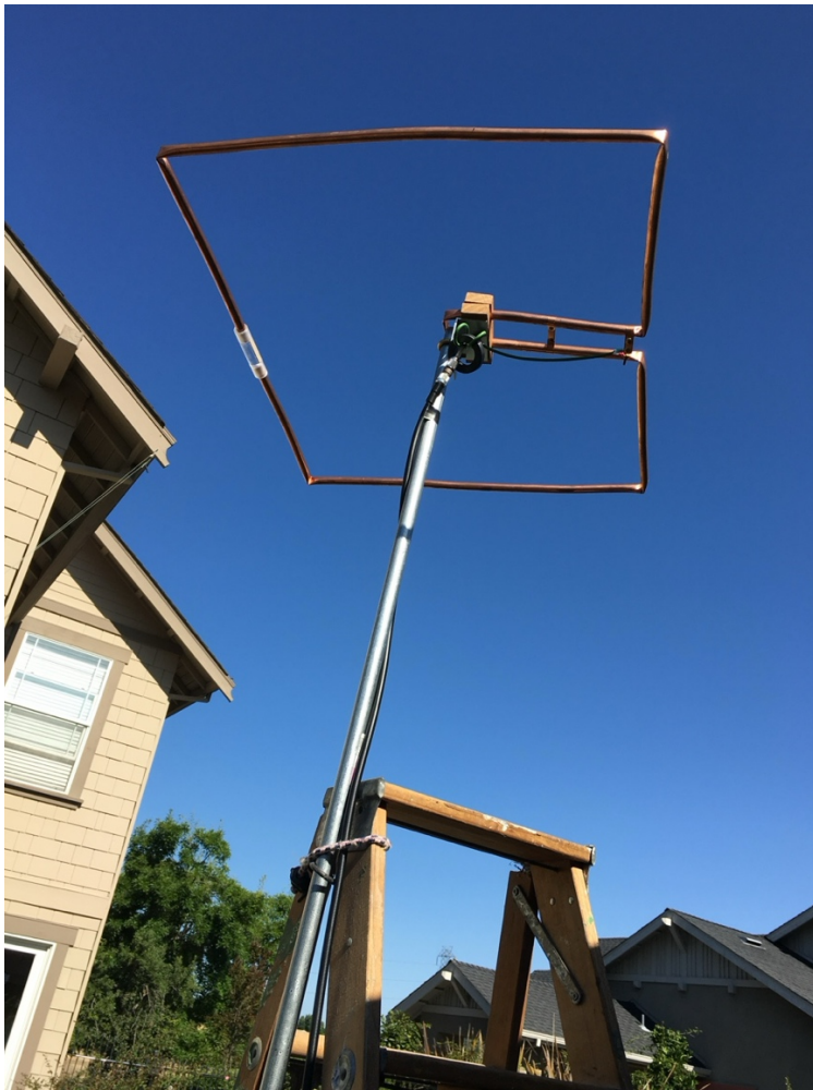
Figure 1. My emergency 6 m squalo, made of refrigerator tubing and installed on a piece of conduit.
