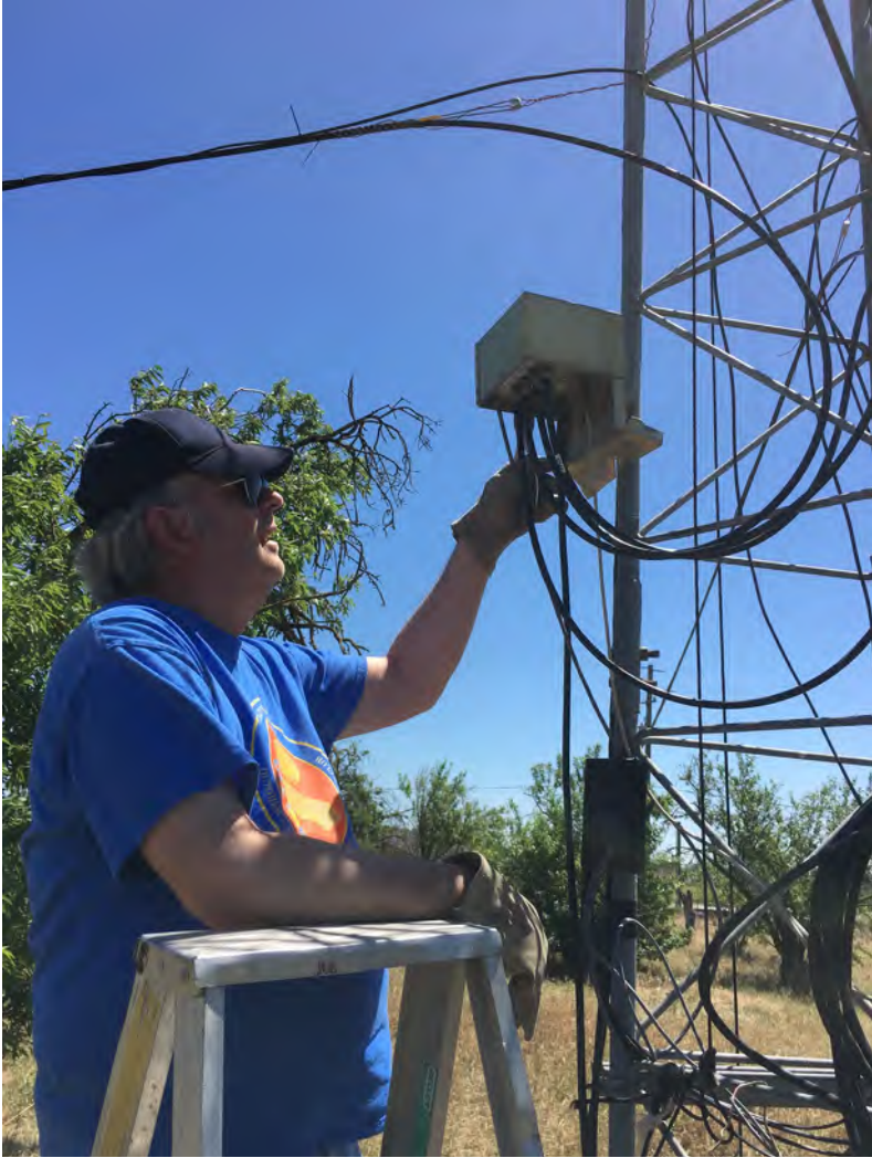
Figure 6. Lee KI6OY tends to the Comtex box. SO-239s get a coat of Dow DC4 dielectric grease, and a good tightening.
