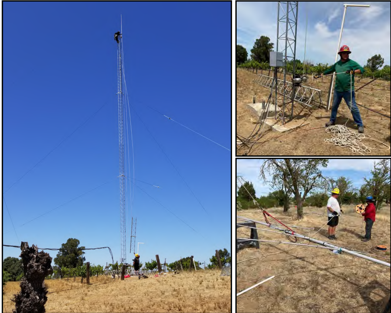
Figure 10. Left, hoisting a tower section. Lower guys are already tensioned. Upper right, the winch operator (KK6PXT) has a lot of responsibility. Lower right, preparing to tram a 10m Yagi.
