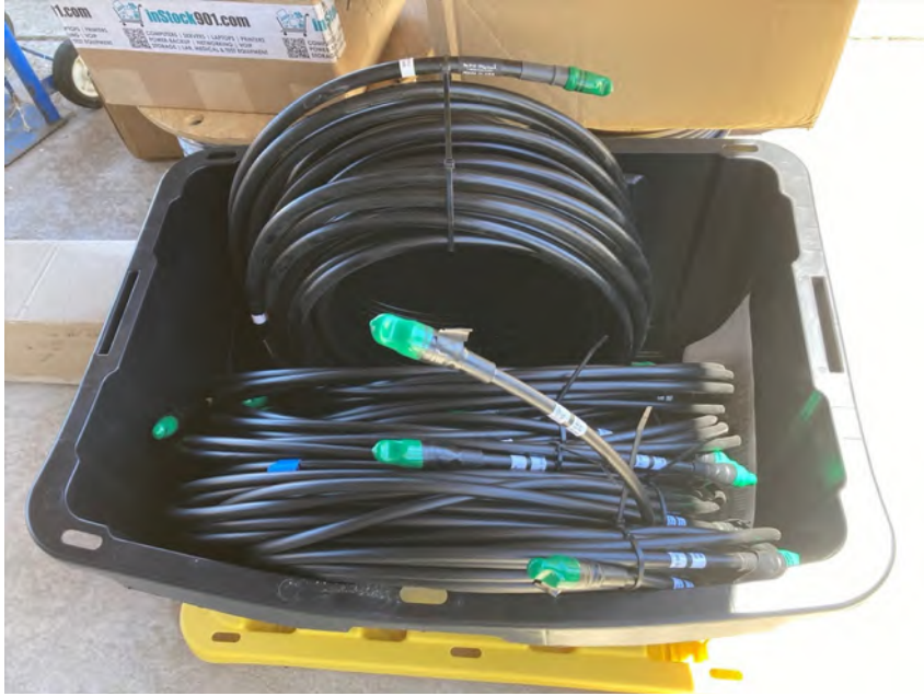
Figure 9. Nearly all the cables ready to go, in one bin. Protected, labelled, and organized.
