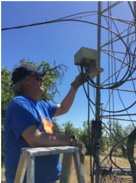
**Figure 7.** Lee tends to the Comtex box. SO-239s get a coat of Dow DC4 dielectric grease, and a good tightening.
