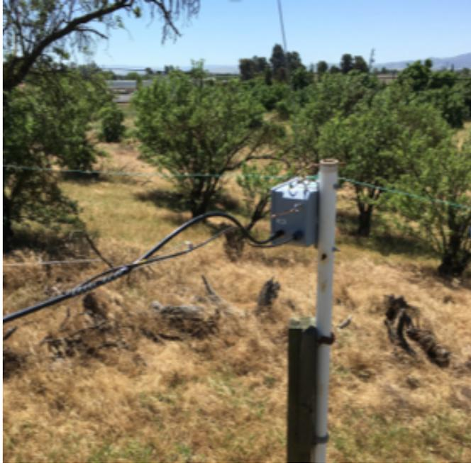
**Figure 5.** Antenna box installed. Feedlines have nice strain reliefs. This should hold up well. If only the wires would survive all that flexing the wind.
