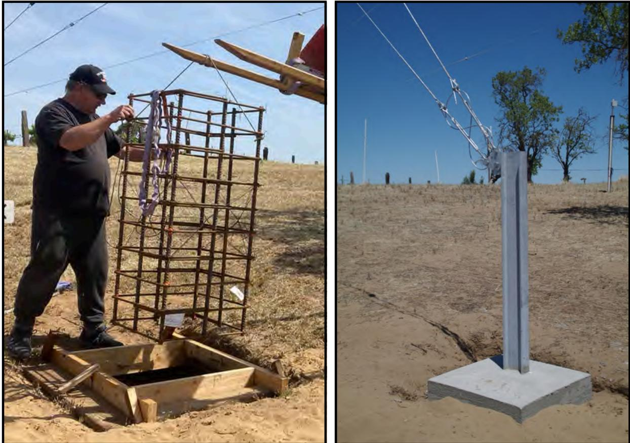
**Figure 5.** New guy anchors have a substantial rebar cage in the base and use galvanized I-beams that are designed to handle the full load with a large safety factor.
