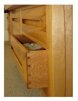
Drawer faces are contoured and dovetailed to oak sides. They fit perfectly in the carcase, with no guides. Handles were routed with a special cutter that I made to allow curved undercuts that fit your fingers nicely.
