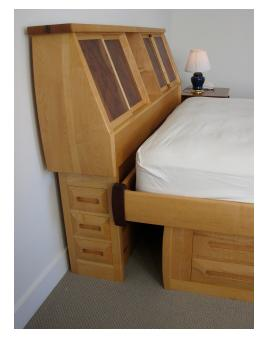
Small drawers are under the headboard, which is a stand-alone unit that is lag-bolted to the bed rail.
